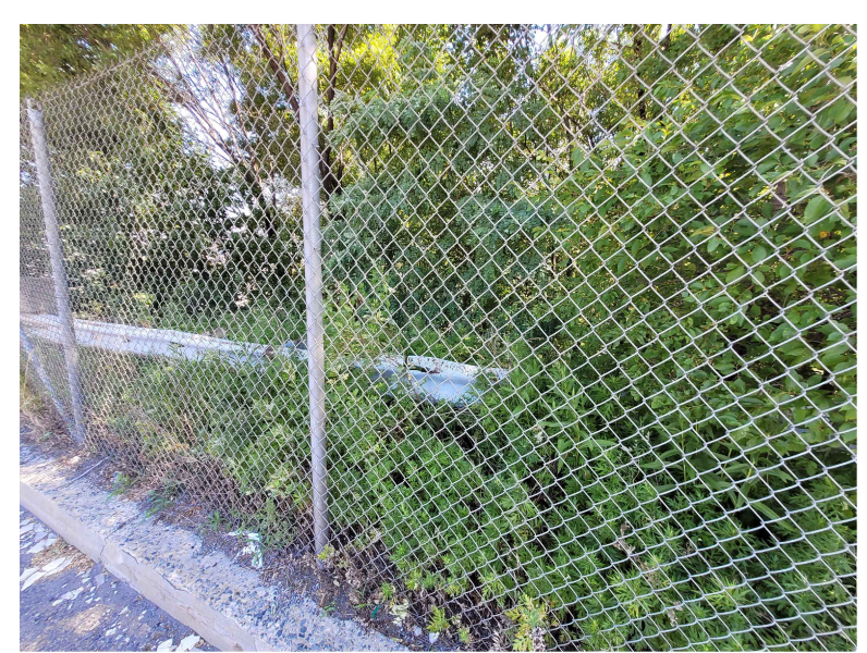
REPLACE THE DAMAGED NORTHEAST APPROACH GUIDERAIL
